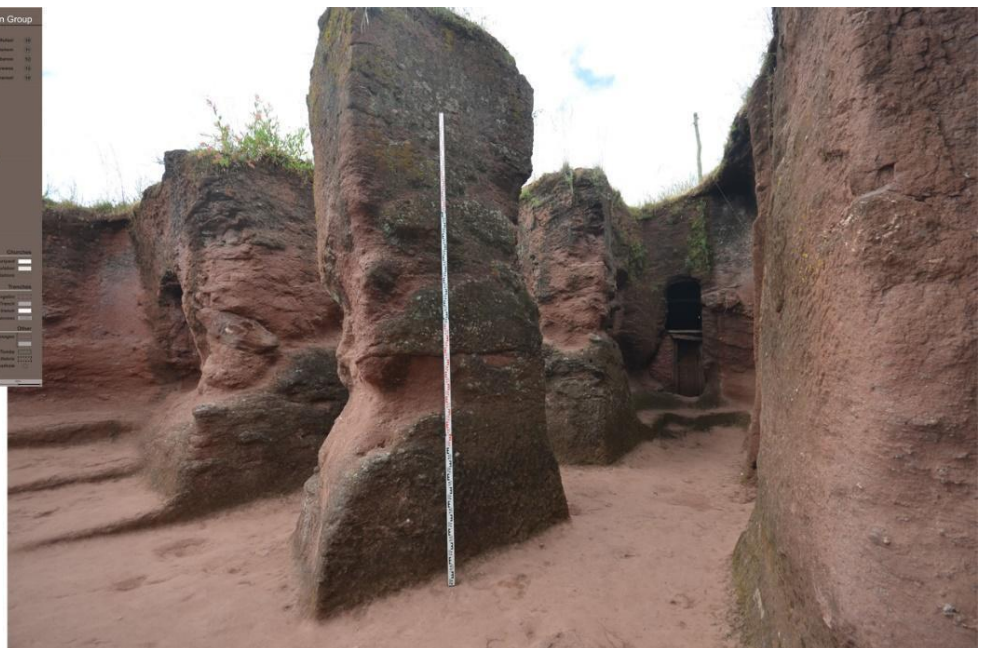
Beta Marqorewos, church on the site of Lalibela. Remains of pillars supporting a completely collapsed rock-cut arch. © mission Lalibela, 2016.
